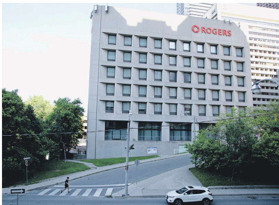
A 54-year-old building at 350 Bloor St. E. in Toronto, owned by Rogers Communications Inc., is slated for demolition and is set to be replaced by a residential tower. ABHIJIT ALKA ANIL / THE GLOBE AND MAIL
